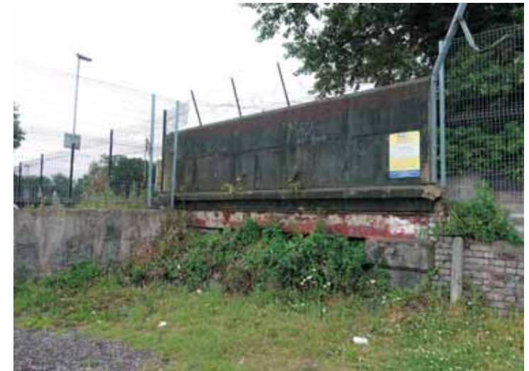
^ Existing bridge remnants of the old canal arm under Jersey Street
